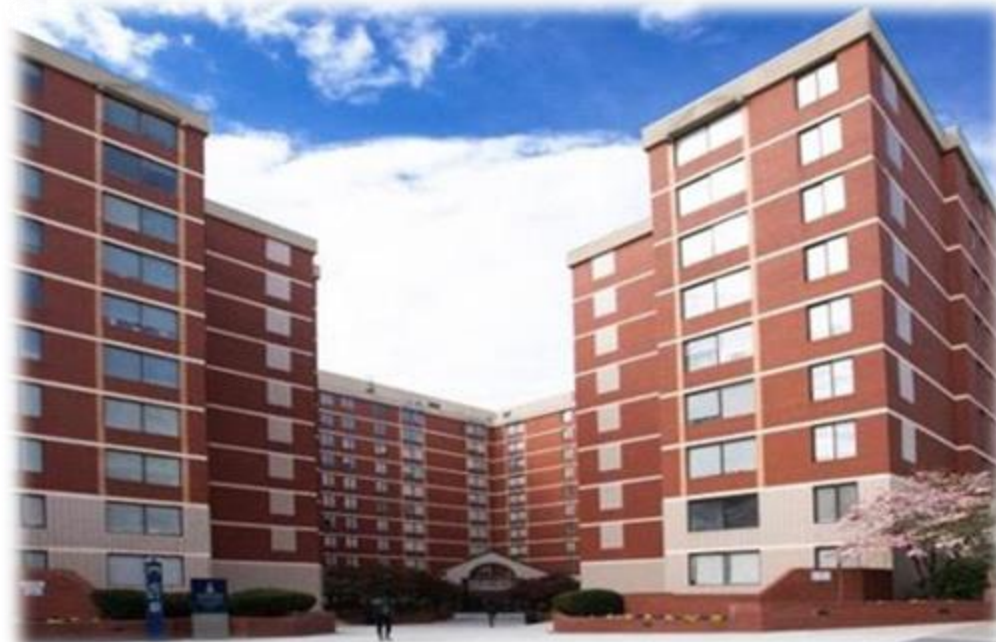
Howard Plaza Towers East and West
